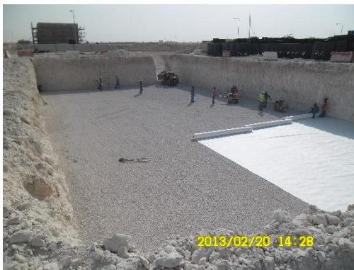
Fig 8: Overlap Geotextile by minimal 12" (300mm) or more. Pull Wrinkles out of Geotextile
