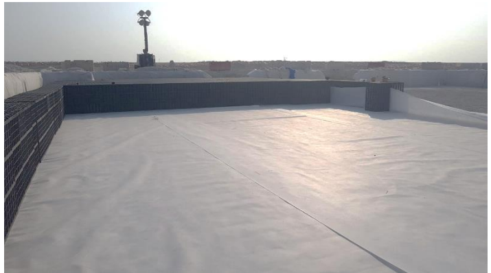
Fig 10A : Place the frame STM tank in Capital "L" format and start building the tank from the corner out to achieve perfect layout.
