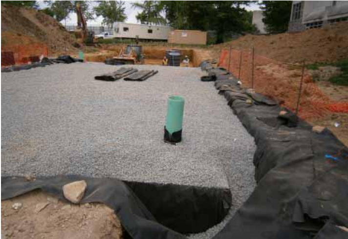
Fig. 17 Use an LGP dozer to push backfill over STM Tank units.
