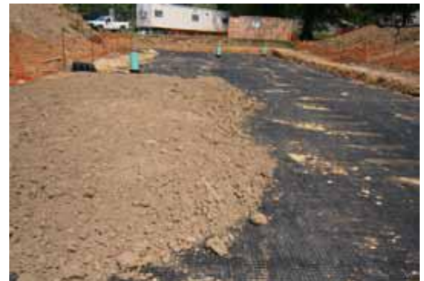
Fig. 19 Pushing backfill parallel to the Geogrid prevents the grid from shoving.
