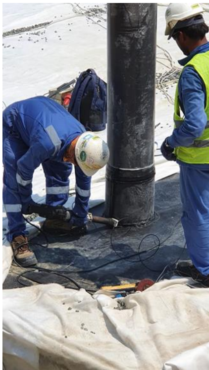
Fig. 11 Cut an "X" into textile to accommodate pipe penetration.
