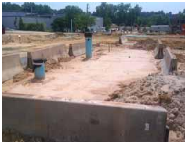
Fig. 21 Secured STM Tank installation using Jersey Barriers.
