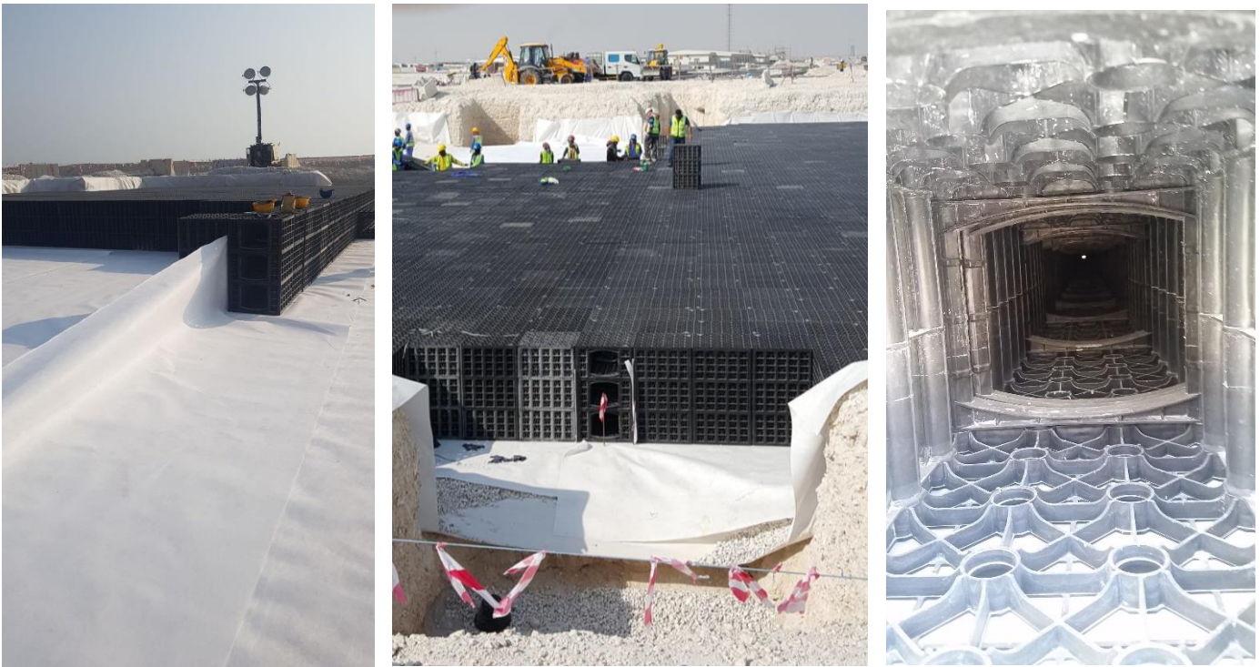
Fig 10 A: Showing Inspection row being installed and being surrounded in its own geotextile casing to prevent debris from spreading into the entire tank Structure.
