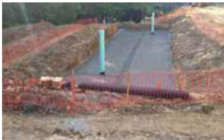
Fig. 20 Secure the installation with temporary fencing.
