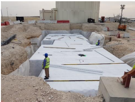
Fig. 12 Encapsulate STM Tanks with geotextile
