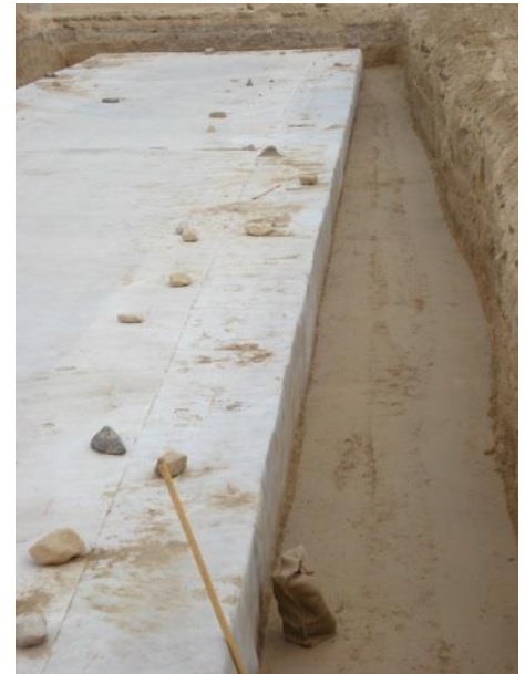
Fig. 16 Vibratory compaction of side backfill is always required , regardless of what backfill material is used.
