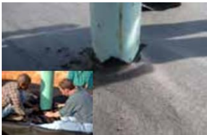
Fig. 11 Cut an "X" into textile to accommodate pipe penetration.
