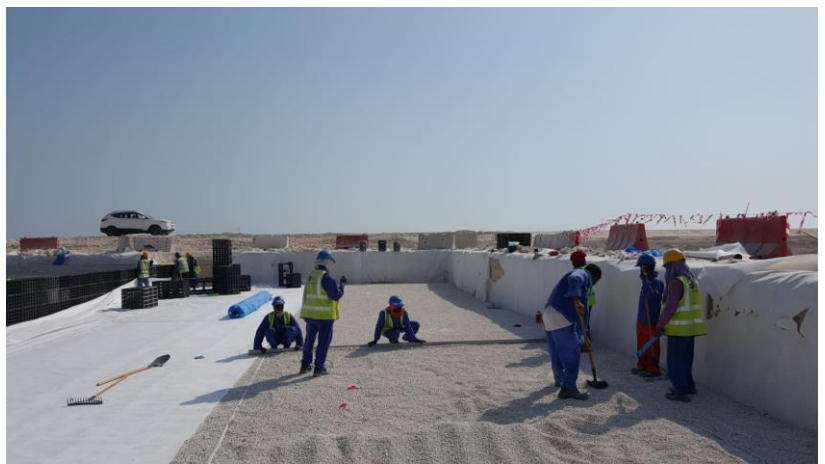
Fig. 3 Compacted and Levelled subbase to 95% proctor
